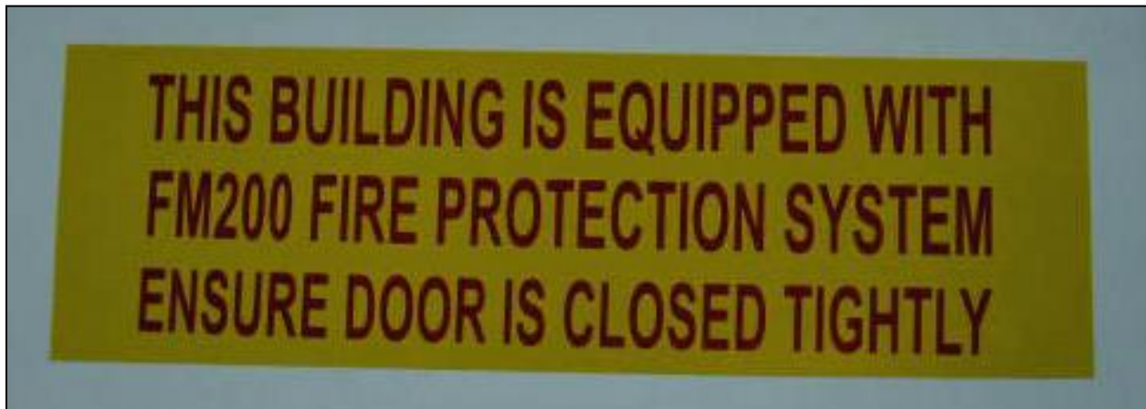
Figure 40: Often electrical switchgear and computer rooms are protected by fire inhibiting gas systems. Typically alarms sound to allow evacuation before such systems are activated. Source: Self-made
